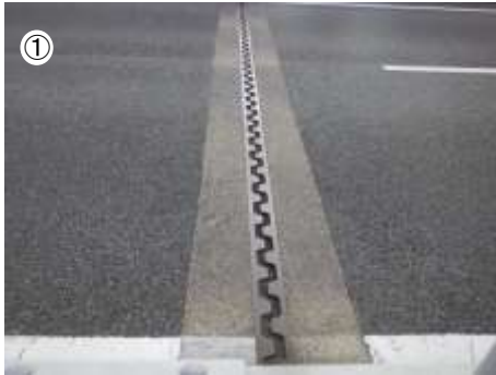
Joint at Root 1. For exchanging seamless joint to remove the steel member.
