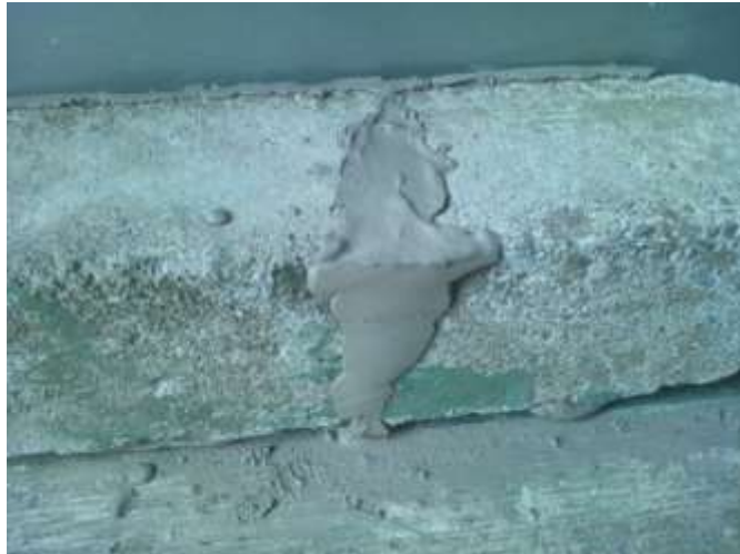
Pouring to cracks.
