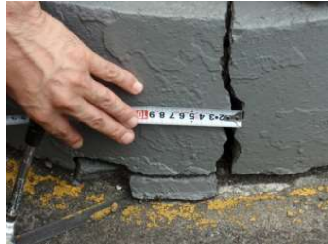
Concrete structure is floating from the floor.
