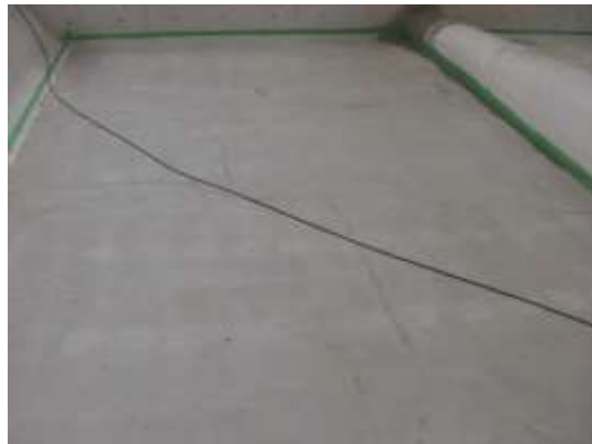
Roughening of the surface and cracks occur in the concrete after curing.
