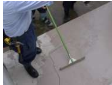
The leveling to 2mm-thick spread with a rubber rake.
