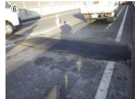
Restored to temporary, full asphalt pavement at a later date.
