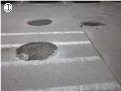
Hole repair test in the rain.
